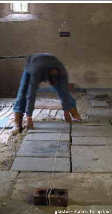
glaster™ Screed being laid
