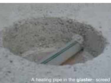
A heating pipe in the glaster™ screed
